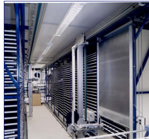
interior view with cooled area
